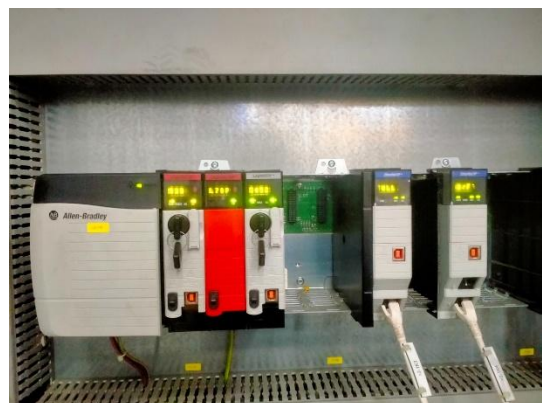
Gambar 1. PLC (Programmable Logic Controller)
